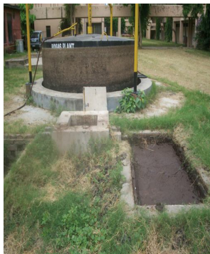
Figure 1. Biogas plant (20 m 3 /d) being fed with jatropha & pongamia oil seed cakes.
